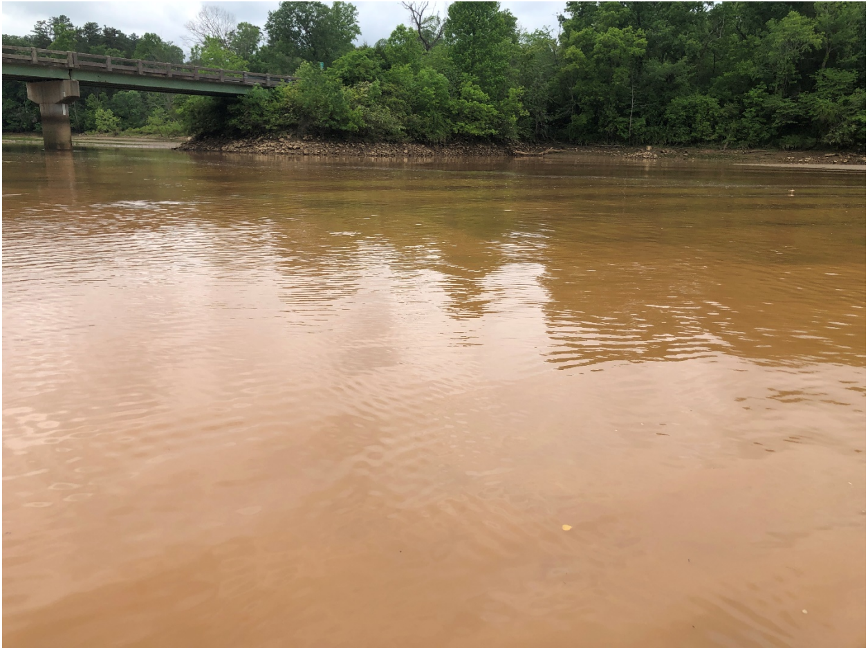
Figure 5 – Water quality observations at Toler Bridge on May 29, 2020.
