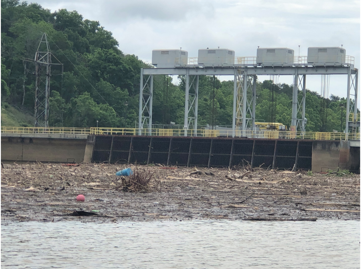
Figure 2 – Buildup of debris at Leesville Lake dam due to heavy rains throughout the area.
