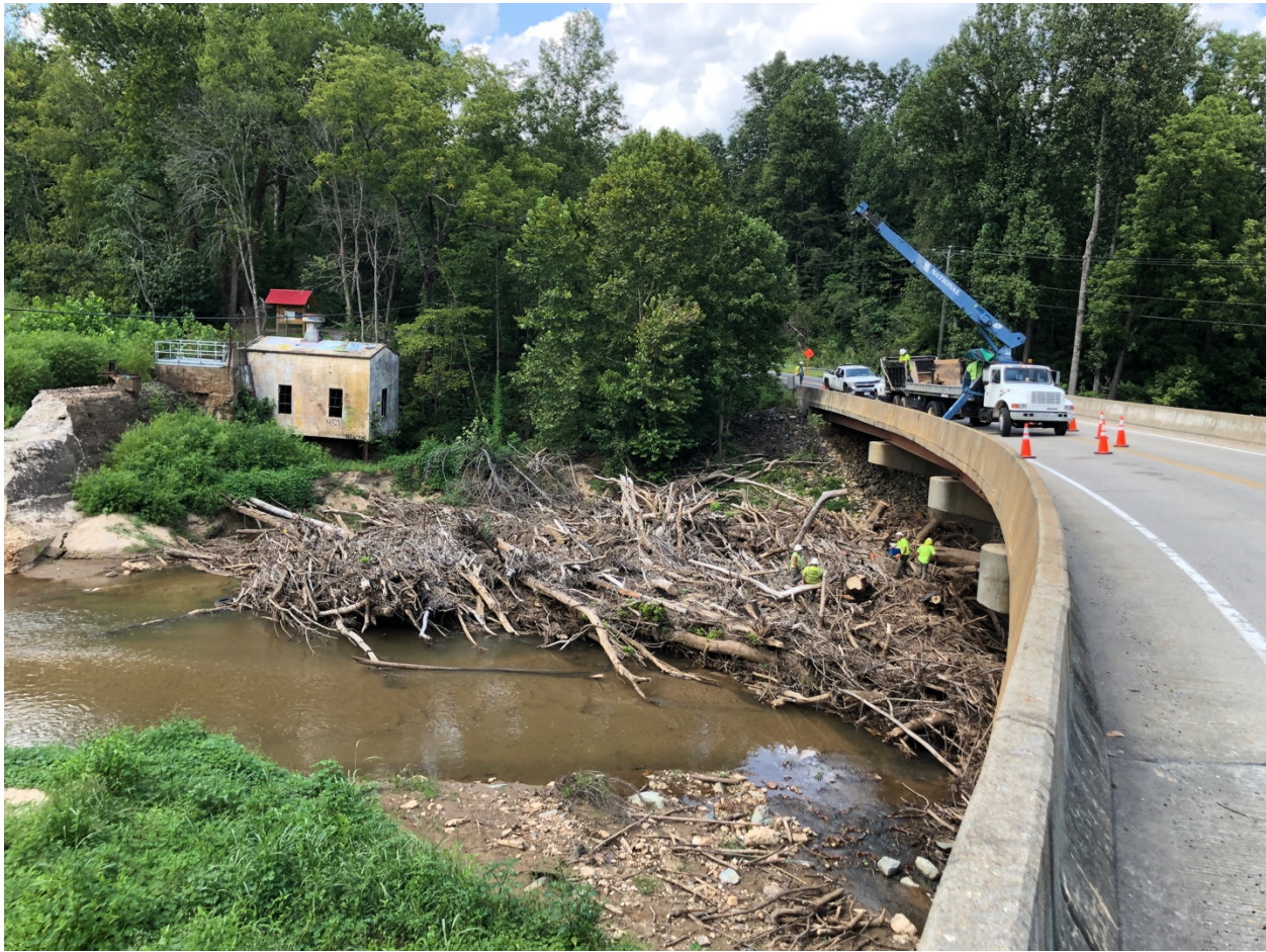
Figure 5 – Excessive buildup of timber from deforestation into bridge on Power Dam Road near Rocky Mount Virginia. Contractors are working to remove the debris (Figure by permission from Author).
