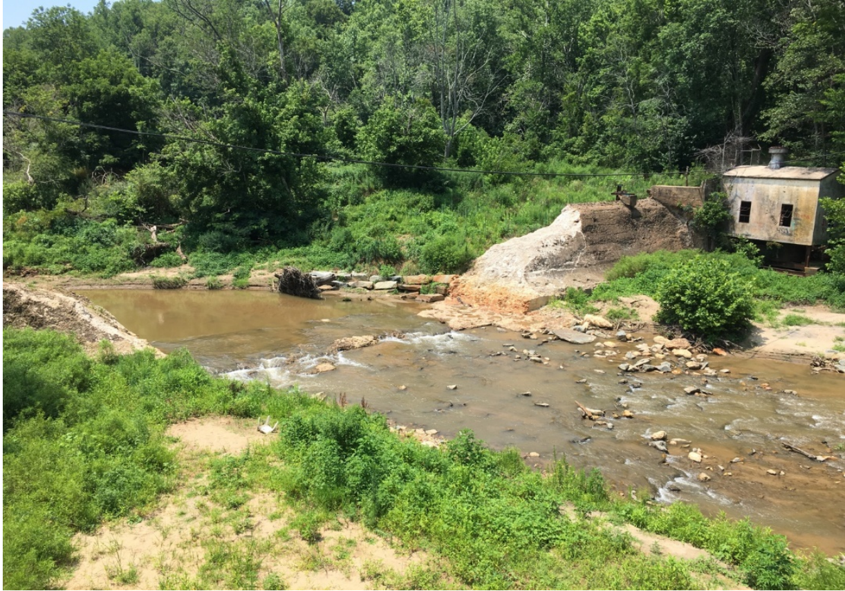
Figure 8- late summer condition of dam on Power Dam Road after removal. Legacy sediment appear to be a continual problem. Note the discoloration of the water even during low flow conditions (Figure by permission from Author).
