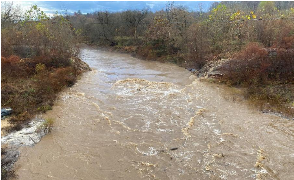
Figure 3.1. Stormwater flowing through old power dam location. Significantly sized debris (branches and logs) can be seen flowing with the stormwater that will eventually enter Leesville Lake.
